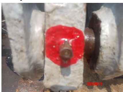
15 May – Before greasing: brake band joint 3
