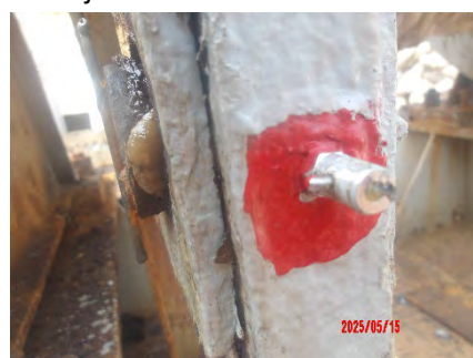
15 May – After greasing: brake band joint 2
