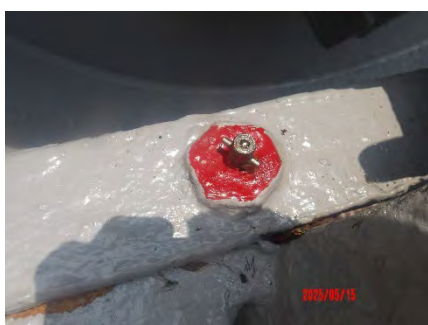
15 May – Before greasing: Clutch handle point
