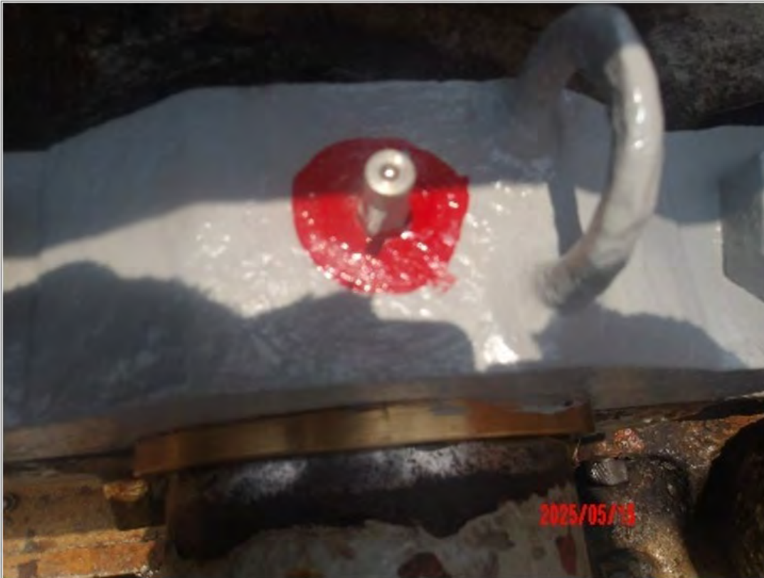
Before greasing of the Bed Frame Bush
