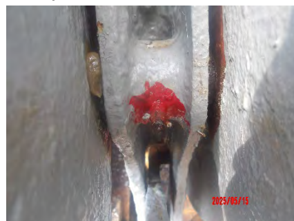
15 May – After greasing: brake band joint 4
