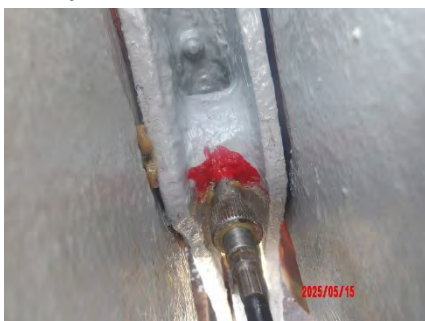
15 May – during greasing: brake band joint 4
