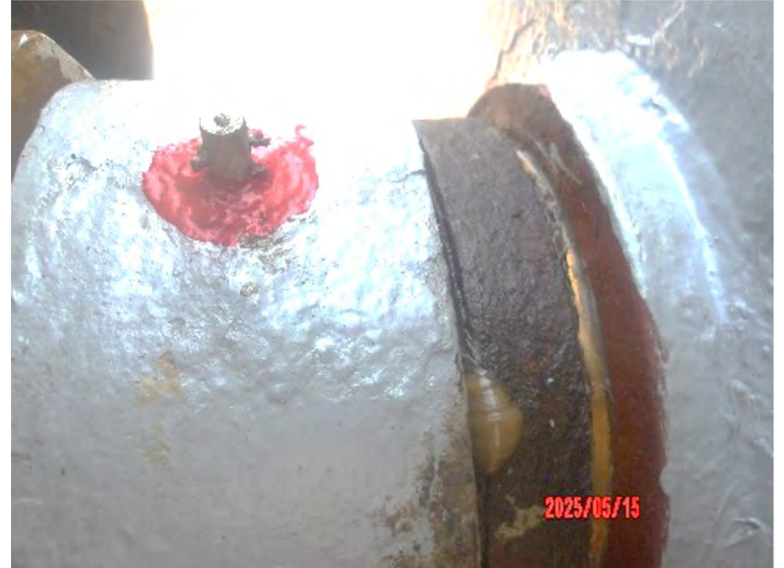
After greasing of the Outer Side Frame
