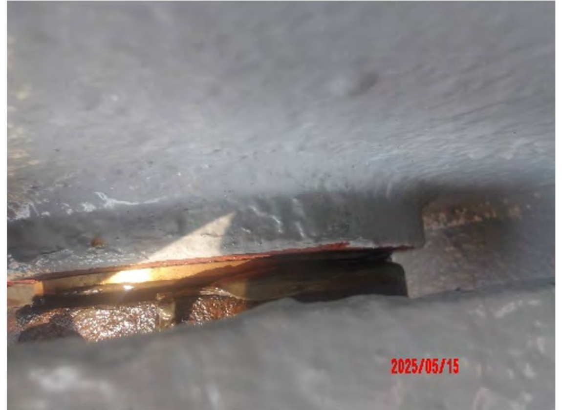
After greasing of the Inner Hawser drum bush
