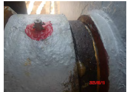
15 May- After greasing: bushing for side frame outer
