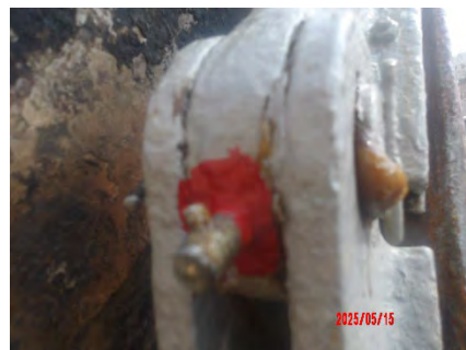
15 May – After greasing: brake band joint 1
