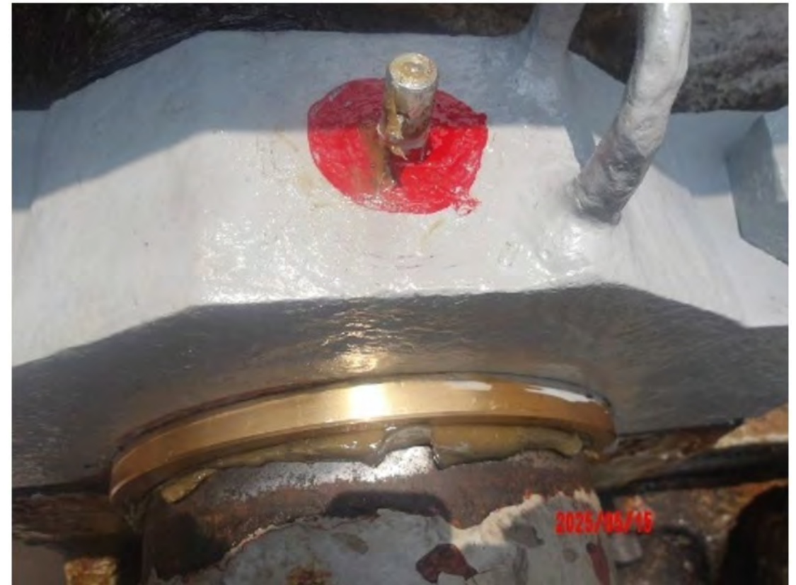
After greasing of the Bed Frame Bush
