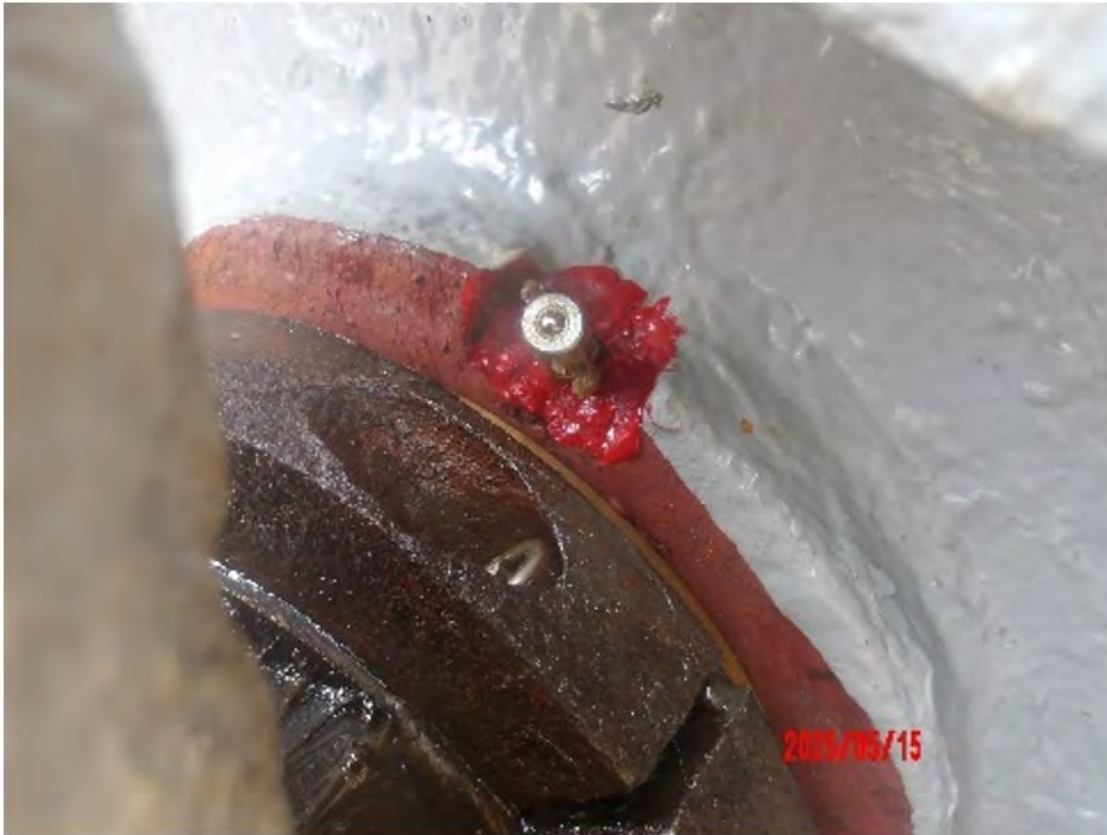
Before greasing of the outer Hawser Drum Bush
